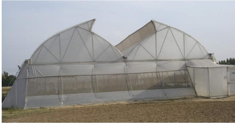
Fig.1 Greenhouse structure having floor area of 560 m 2
