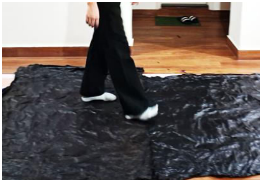
Figure.1 (c) Covered all the layers with plastic sheets and press firmly by walking over.
