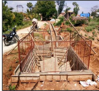
Fig.1 Construction of Type-I Injection Wells
