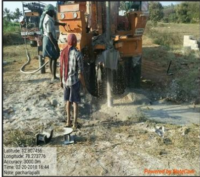
Fig.1 Construction of Type-I Injection Wells
