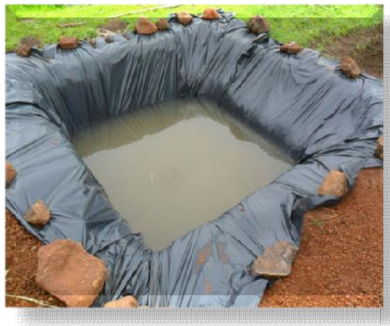
Fig.2 In-situ water conservation in silvo-pasture system through Jal-kund
